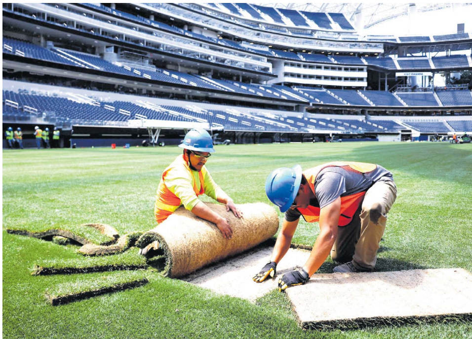
Workers install a patch of grass to be used as part of the pitch at SoFi Stadium, ahead of the FIFA World Cup soccer tournament, in Inglewood, California, U.S., May 13, 2026.
